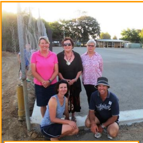
The very happy Terip Tennis Club Committee, Frances Lawrence, Helen McKenzie, Sue Martin, Cindy & Tim Hayes are looking forward to the completion and opening of the resurfaced Terip Tennis courts.
