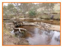
Around 50 structures were installed throughout the three work trial sites, including an additional two log jam constrictions between sites 1 and 2.
