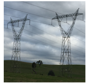
Main north - south Dederang transmission lines. The proposed Molesworth, Caveat, Highlands transmission lines will be similar lattice structures
