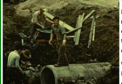
First in went the culverts! Then a mosquito fleet of farm tractors dug and moved the clay and gravel road-base material into position, before the work of levelling and flattening it out was conducted. Images in this article were taken from an old Victorian Country Roads Board film, which shows in good detail some of the road works in progress. That film is now publicly available.
